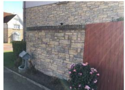
Photograph No. 12 Curved wall at 18 Seaview Avenue
