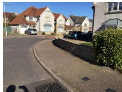
Photograph No. 11 Wall at 1 Seaview Close
